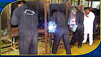
Welding & Fabrication Trade
